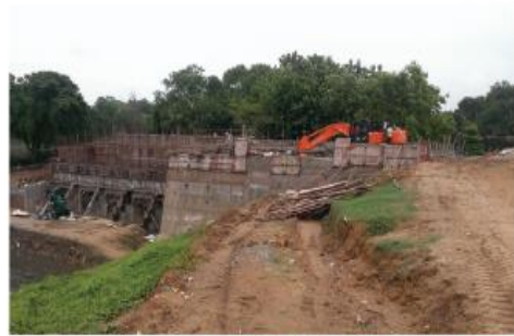
Pumping Station at Binakhandi Work in Progress
